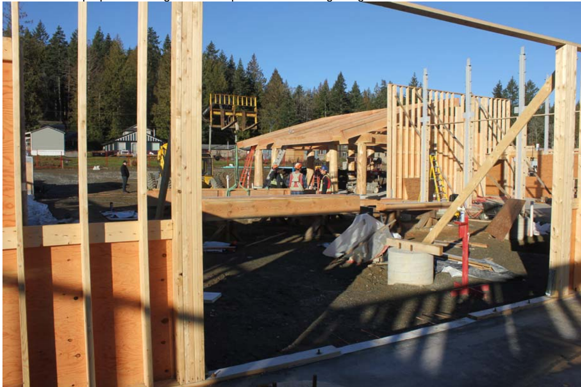
Photo 17: Multipurpose building: 6x6 wood posts at entrance glazing
