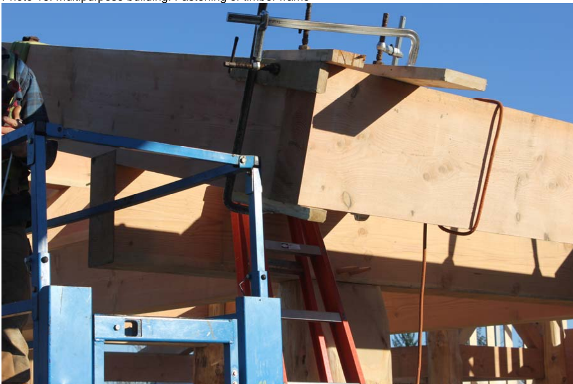
Photo 16: Multipurpose building: Fastening of timber frame
