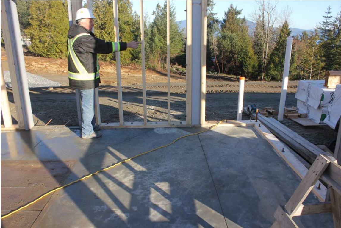
Photo 12: Recreation Centre: North wall: wood framing and steel columns
