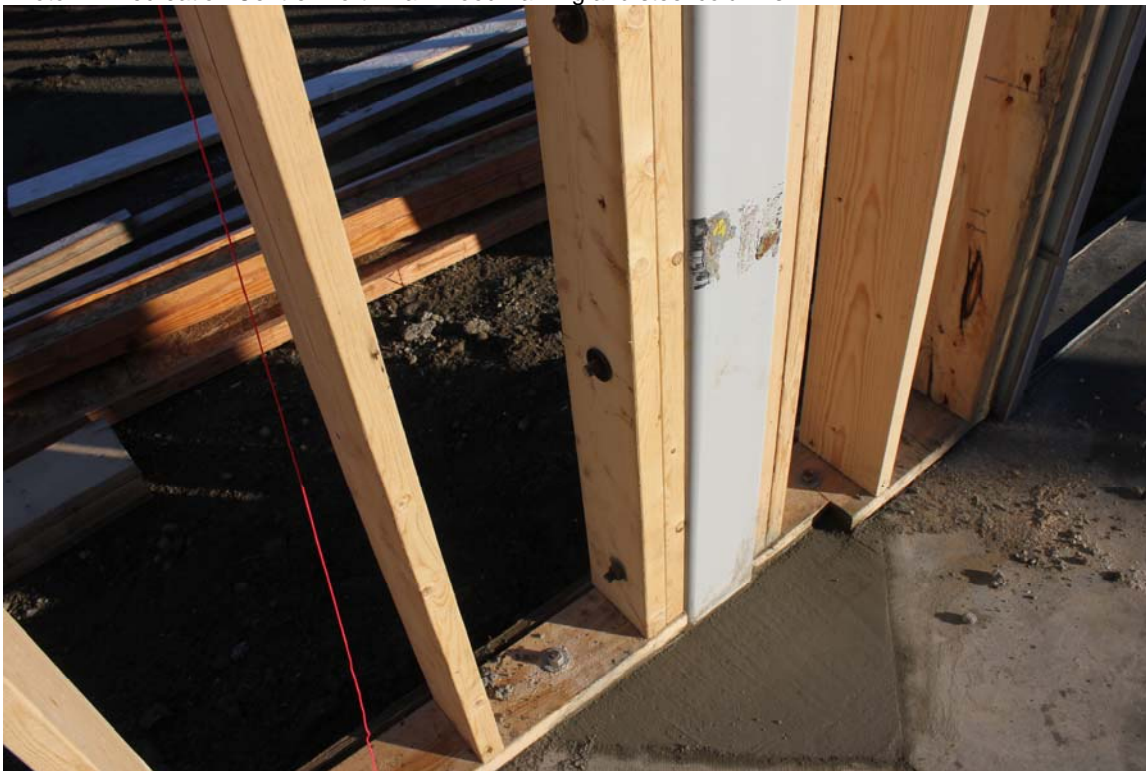
Photo 12: Recreation Centre: North wall: wood framing and steel columns
