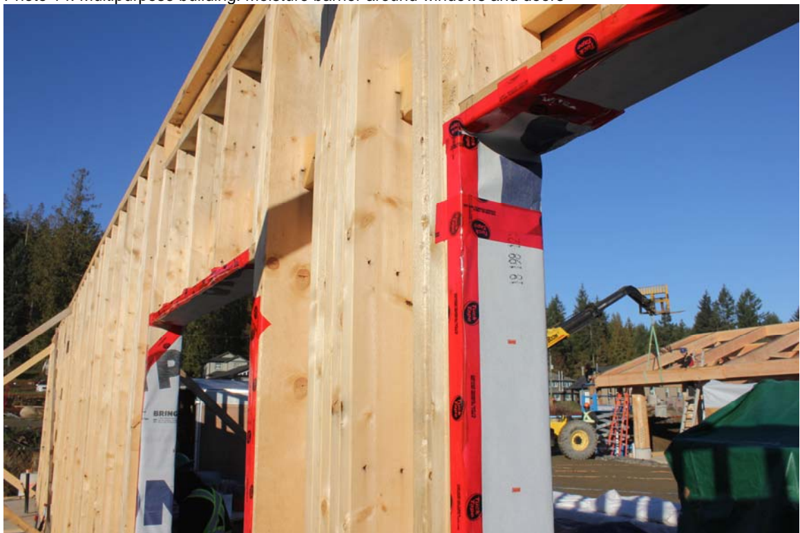
Photo 14: Multipurpose building: Moisture barrier around windows and doors
