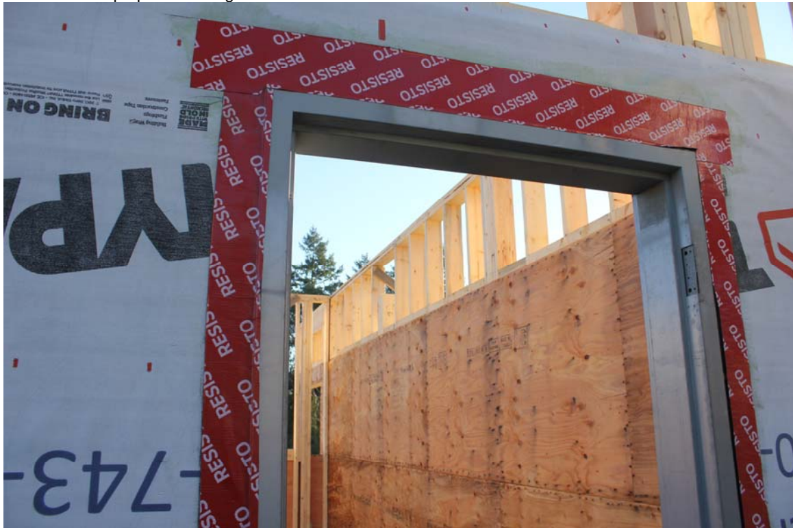
Photo 14: Multipurpose building: Moisture barrier around windows and doors
